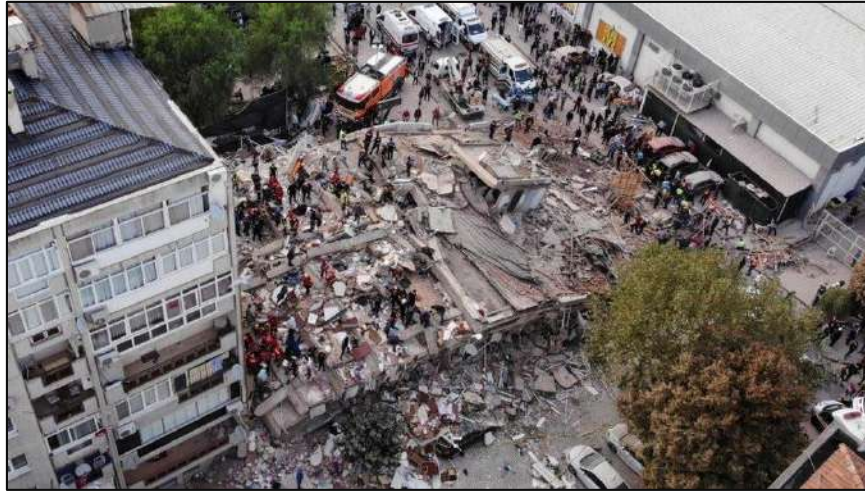
Figure: Vertically damage of a building
