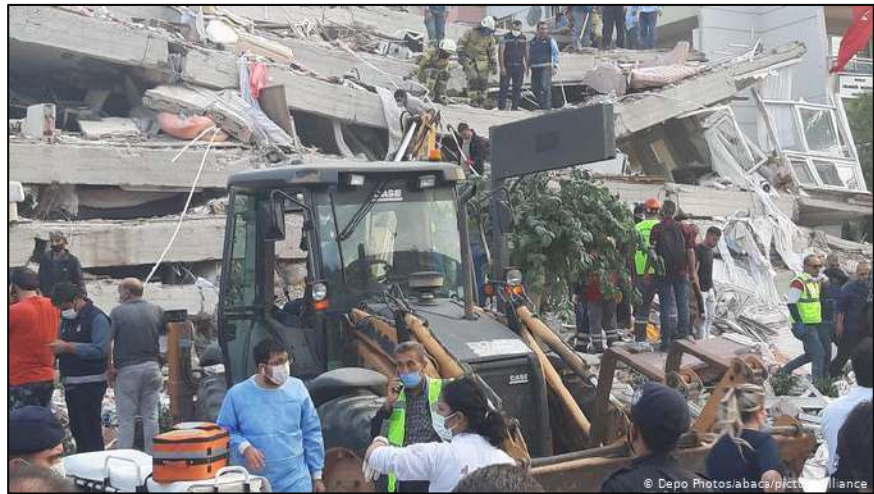
Figure: Collapse of a building
