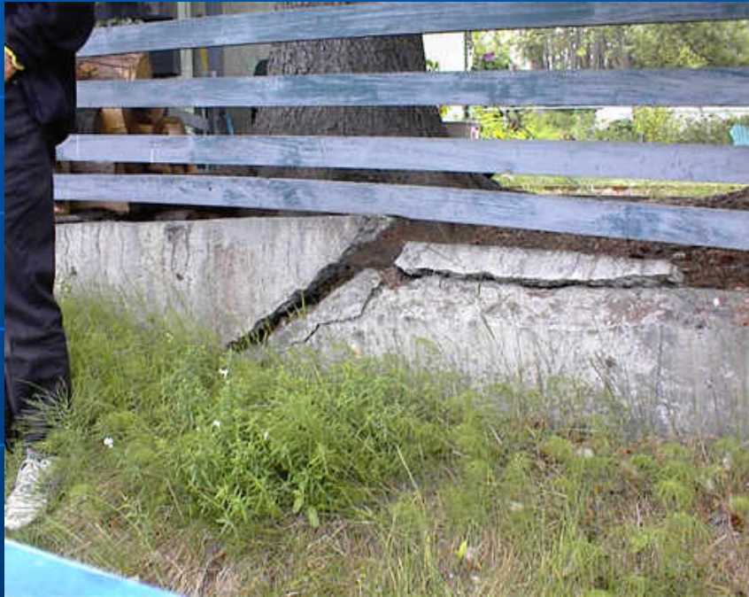
Thrust Fault in Concrete from 1964 Quake, Anchorage, Alaska www.ucmp.berkeley.edu/.../alaska/0709log.html
